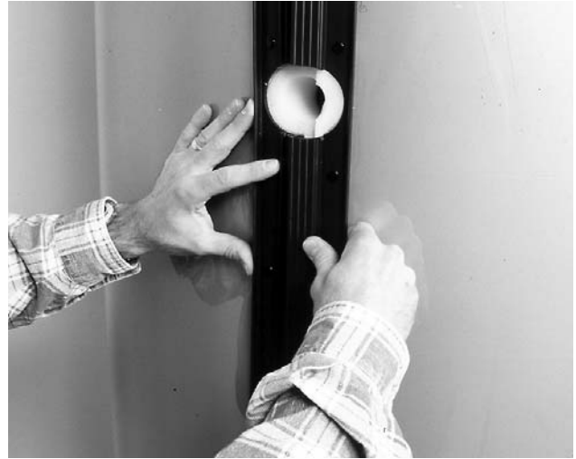
Figure 2 Remove protective transport film and wrapper, remove insulation of RATIO HP 500 by opening the hook closure and set aside to prevent damage to the insulation.
