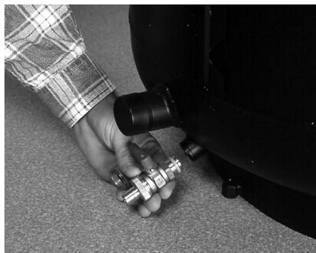
Figure 4 Connect filling/emptying cock at the bottom of the buffer cylinder. Use 5/4" connection in upper, dished end of tank, e.g. filling/emptying cock with reduction or cap.
