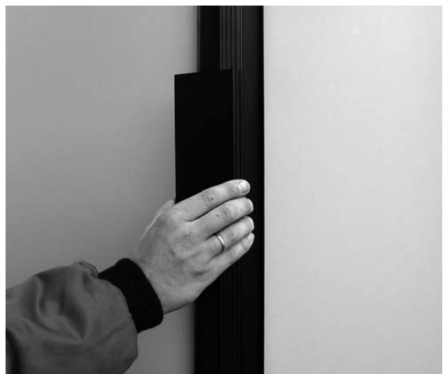
Figure 12 Then close the rear hook closure (opposite to the connections) of the jacket insulation. This may require the use of an assembly tool (Art. No. 130 00 239) or secure hook strip into place with screws.
