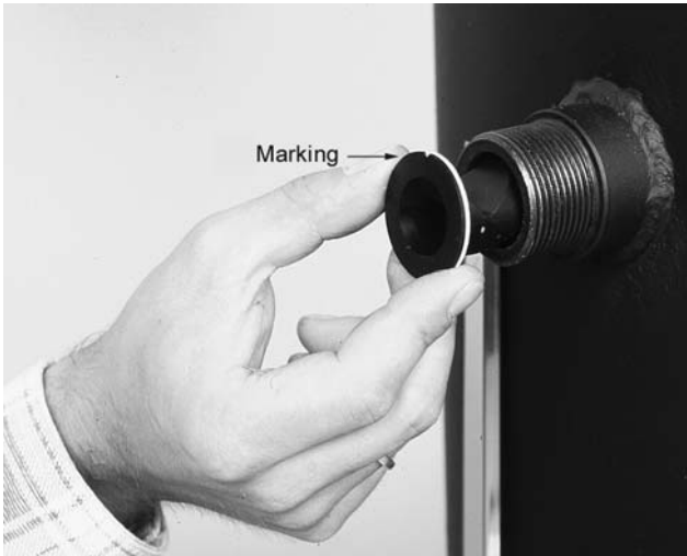
Figure 5 When installing the convection brakes (part of the buffer cylinder connection kit), please consult the assembly instructions included with the kit.
