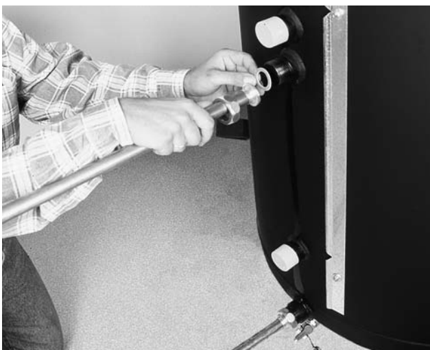
Figure 8 In case of buffer cylinder with solar heat exchanger: Connect solar circuit with heat exchanger (flow and return). The inlet into the solar circuit heat exchanger is at the top and the outlet at the bottom.
