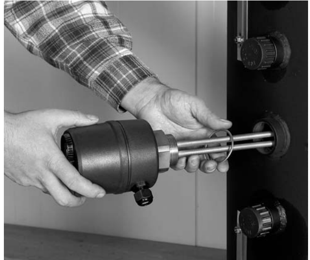
Figure 10 Option: If needed, install electrical auxiliary heating. Please consult the information included with the immersion heater to ensure the auxiliary heater is installed correctly.
