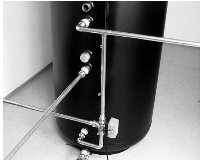
Figure 7 When integrating the solar installation into the heating system using a return flow increase, please use the optional switching valve kit (Art. No. 130 100 19).
