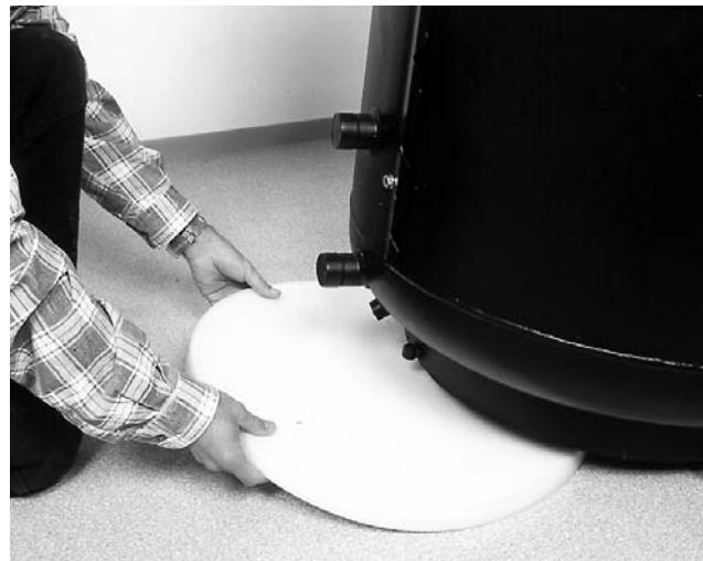
Figure 3 Unscrew cylinder from pallet and transport to the installation site (weight up to 205 kg!) Turn cylinder so that connections point towards installation wall, tilt and insert inner section of the floor insulation.
