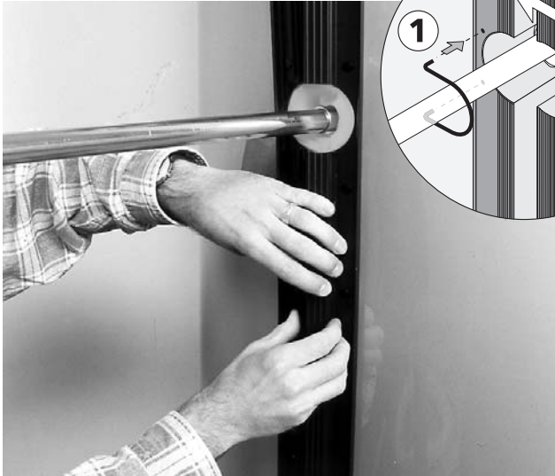
Figure 13 Close insulation with front hook closure. First snap into the weakest groove position and then alternately retighten.
