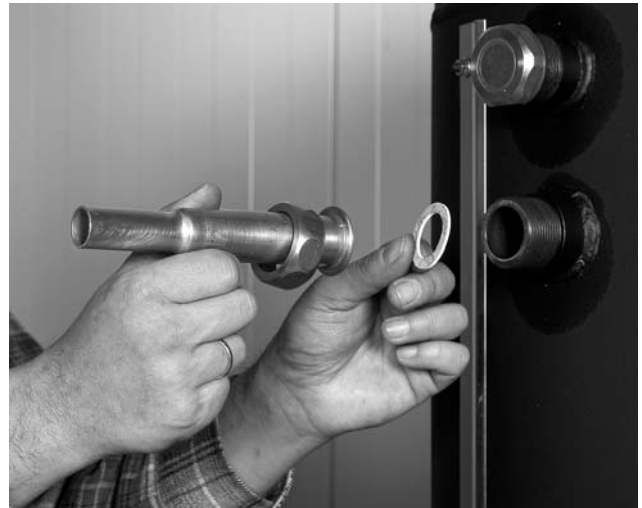
Figure 6 Depending on system solution, connect heating connection pipes with buffer cylinder using flat seals. Cap unused buffer cylinder connections with 5/4" caps.
